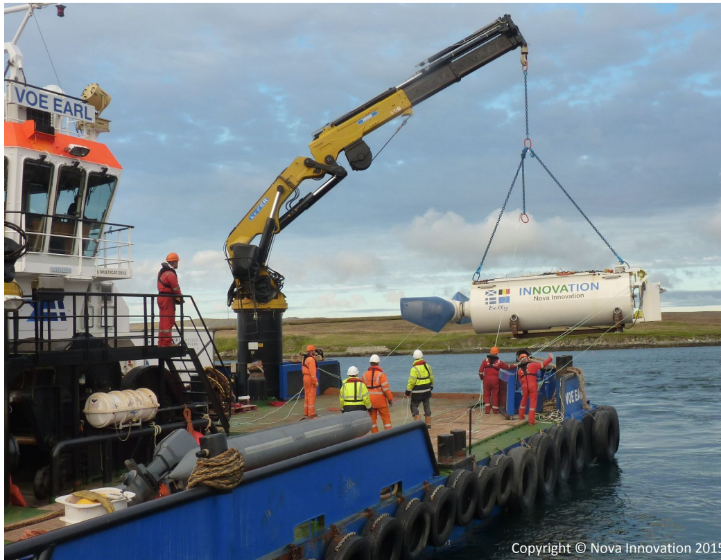
Figure 9: Nova M100 Installation at Bluemull Sound Site 11
